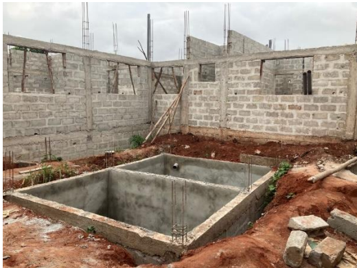
Construction of the Medical Clinic
